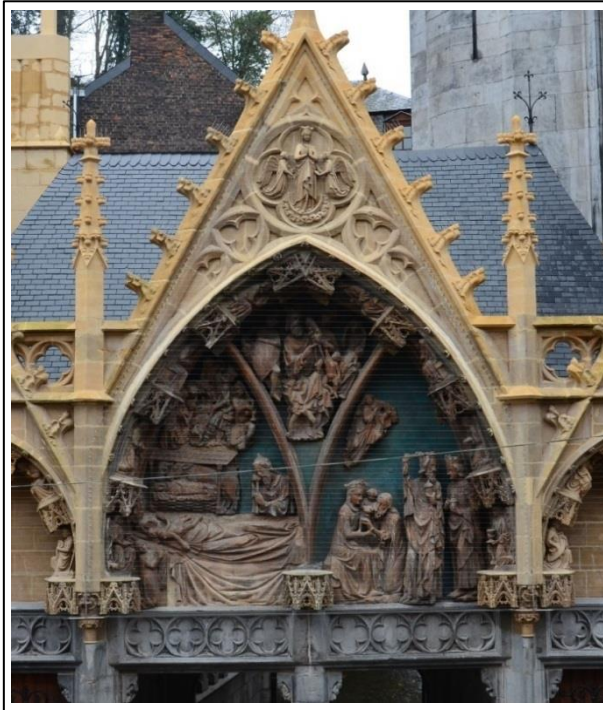
Fig. 8: Portal after maintenance treatment in 2014.
