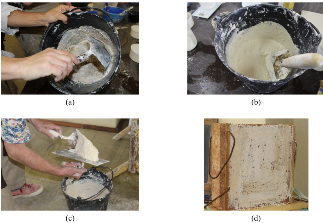
Figure 2.16 - First layer of a multi-coat plastering system: (a) mixing lime and sand; (b) and (c) lime mortar, ready to be applied; (d) rammed earth substrate after application of the first layer
