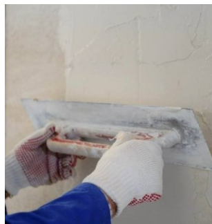
Figure 2.18 - Finishing layer: application of the lime-gypsum paste over the regularization layer
