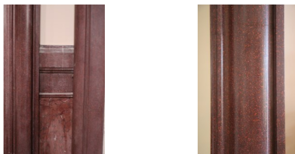
Figure 4.113 - Estoi Palace: plaster decorative elements simulating imperial red porphyry in the Noble room
