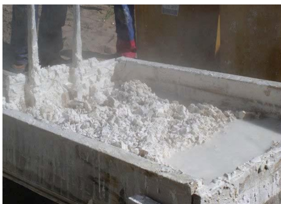
Figure 5 Process of lime slaking
