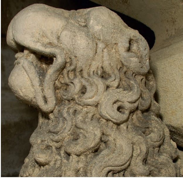
[19] Stone monument with acute decohesion and deposited dirt before treatment.
