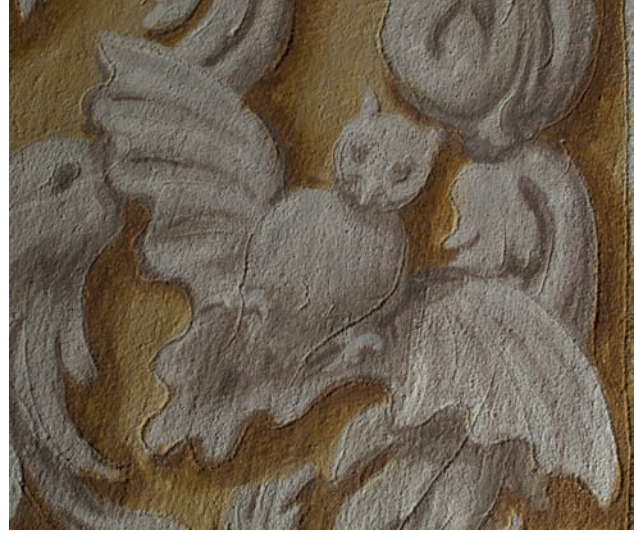
[18] The same area as Fig. 17, after removal of non-original materials.
