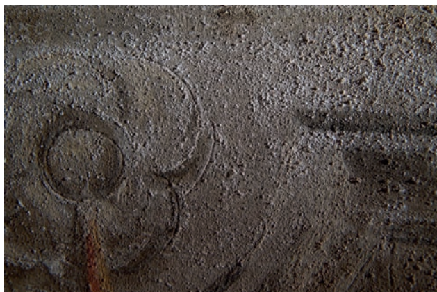
[15] Detail of salt efflorescences on painting, photograph taken during prevailing (baseline) environmental conditions (June 2003).
