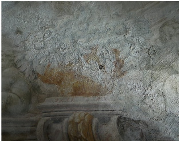
[9] Most of the paintings were covered in a heterogeneous white veil of salt efflorescences and biofilm. The salt activity disrupted the paint layer and the biofilm obscured much of the painting.
