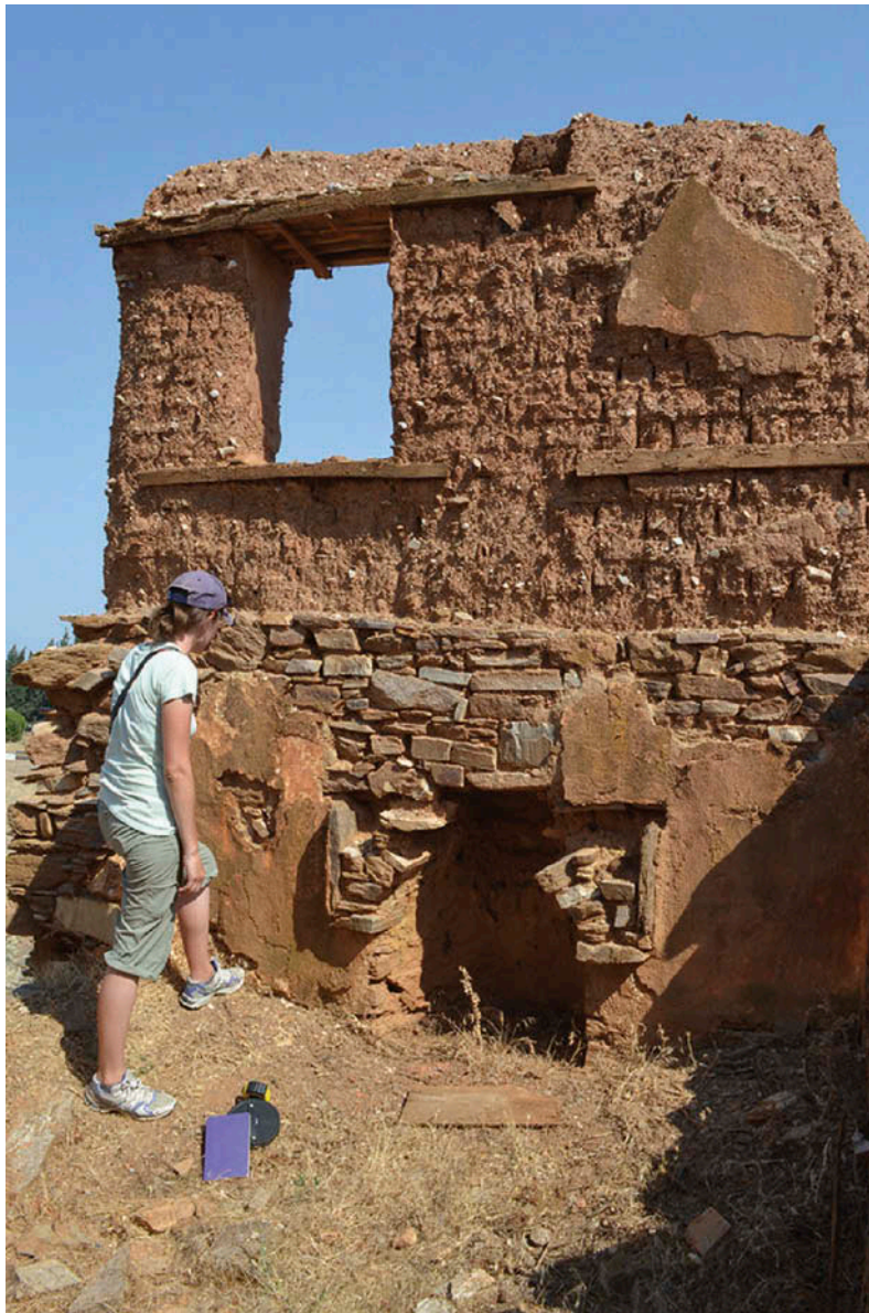
Figure 4. Typical vernacular mudbrick architecture where mudbrick is laid across stone foundations and wood beams provide support; please note areas where original plaster surfaces are preserved, Eski Haciveliler.
