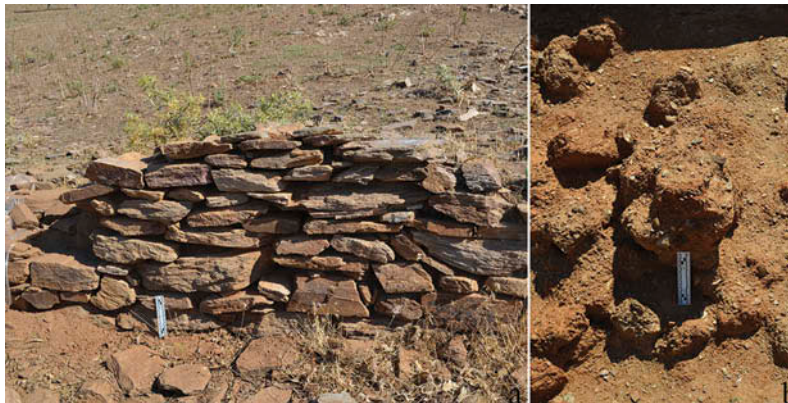
Figure 5. Eski Haciveliler conservation laboratory testing sites: (a) fieldstone masonry wall (south side) surrounding the schoolhouse perimeter and (b) mudbrick wall (west side) from the schoolhouse.
