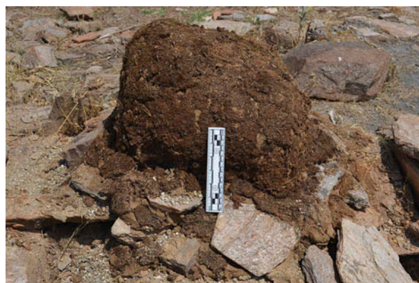
Figure 7. Soft vegetative cap applied to vertical and sloped surfaces of mudbrick (north side) at Eski Haciveliler.
