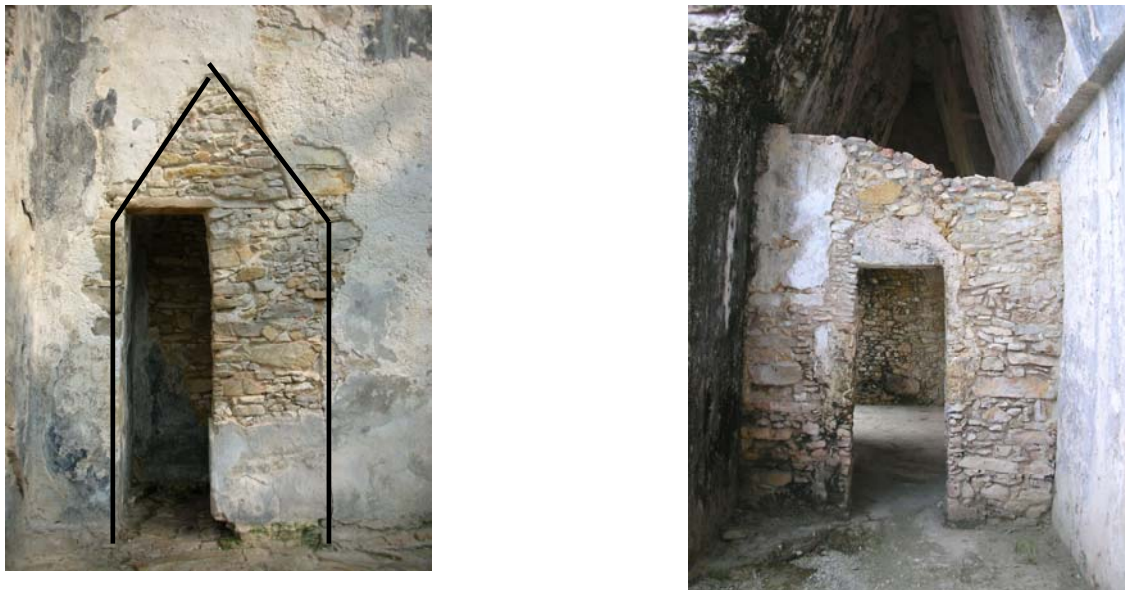
Fig. 7.2. Architectural modifications. Left: modification of a doorway at the Temple of the Foliated Cross with partially lost mud plaster. The orange line shows the original shape of the doorway. Right: dividing wall in the House D of the Palace.
