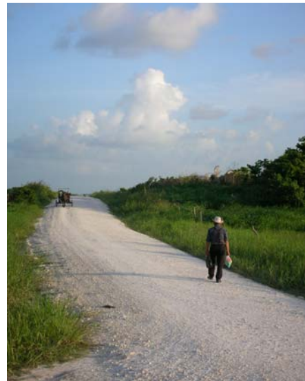
Fig. 7.23. Construction of sascab roads in Belize, close to the site of Lamanai.
