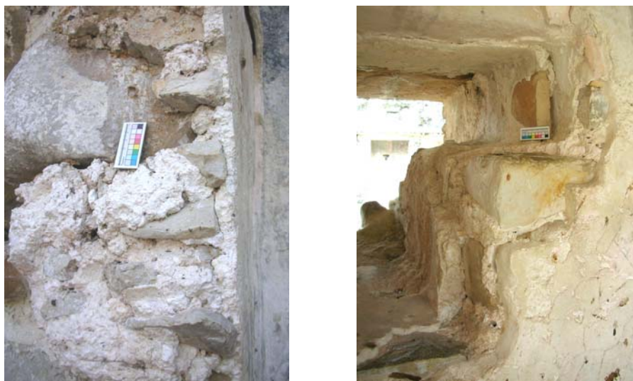
Fig 7.4. Thick pure lime plasters used as joining mortars and renders. Left: original wall at Temple of the Foliated Cross (cross section of collapsed wall). Right: original wall in House D of the Palace.
