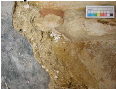
Fig. 7.3. Dividing wall (architectural modification) at the Temple of the Foliated Cross. Mud plaster with unmixed lime lumps. A limewash painted on black can be seen at the left.
