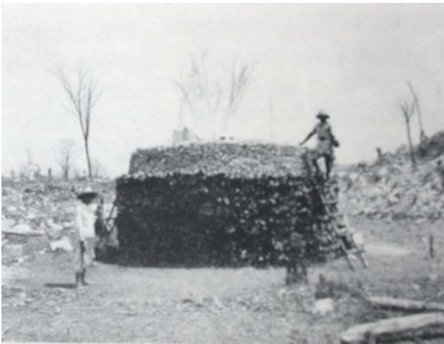
Fig. 3.4. Left: Calera construction in the early 20 th at Chichén Itzá. Right: After the burn the lime is left to slake in the open air. Pictures: Morris and colleagues (1931).
