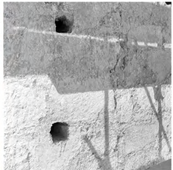
Remains of a wooden cross-bar in a putlog hole (left), Church of St. Lawrence, Požega (Croatia), late 13. century; Photo: 1993, HRZ (Ivan Srša); open putlog holes in a wall (top right) and detail (bottom right), Church of The Blessed Virgin of the Rosary, Remetinec (near Novi Marof), second half of 15th century; Photo: 1992, HRZ (Ivan Srša)
