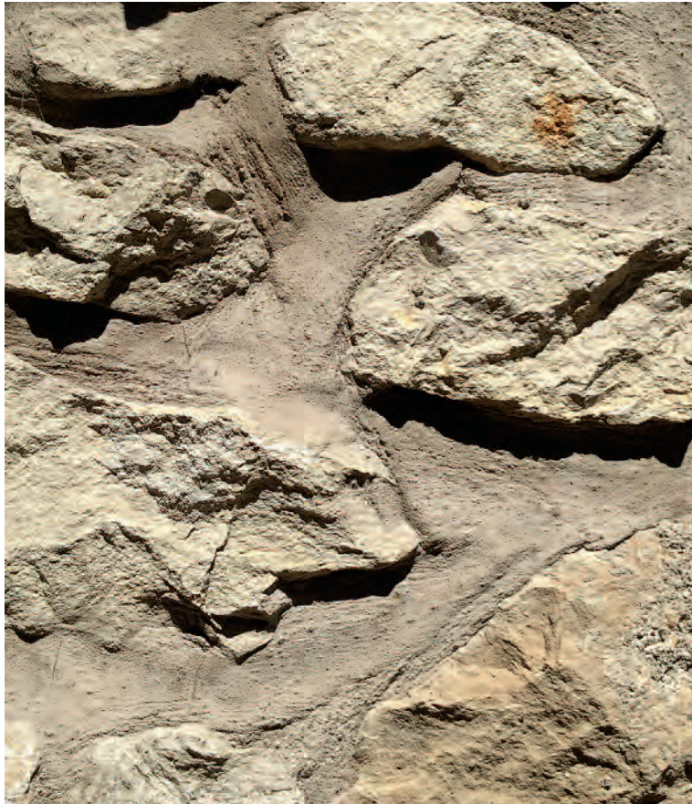
Natural stone masonry joint, Safranbolu (Turkey), 19th century; Photo: 2014, KBU (Aysun Özköse); Illustration: 2015, Raimar Heber based on a drawing by Oana Gui
