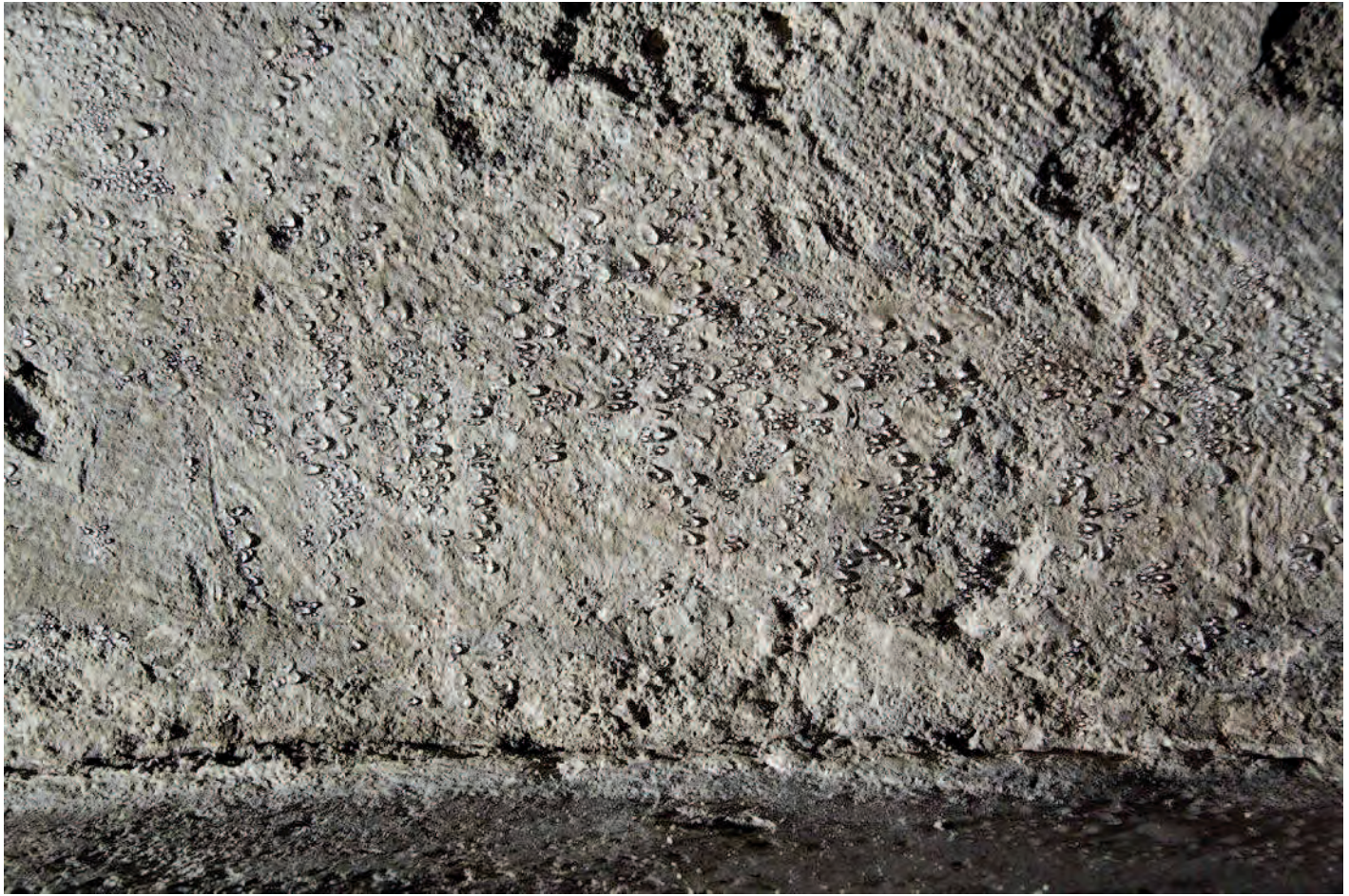
Water droplets condensing on a surface, St. Georg, Reichenau-Oberzell (Germany); Photo: 2012, RPS (Dörthe Jakobs)
