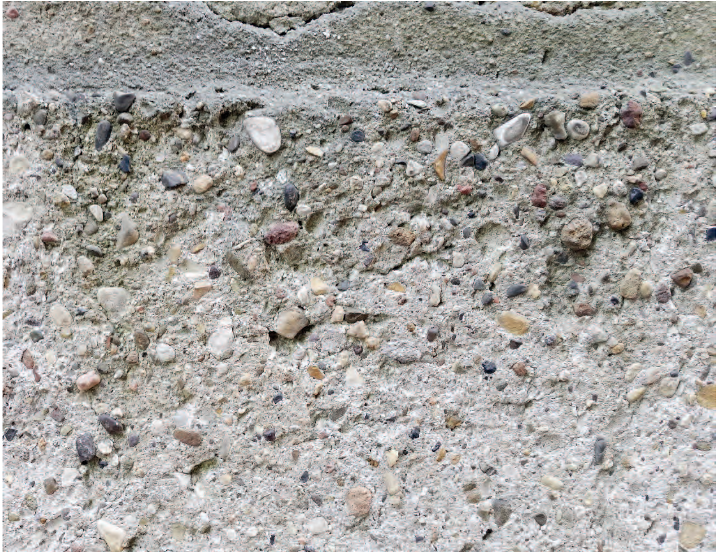
Detail of rough cast finish on an exterior wall, private building (detail), Hildesheim (Germany), mid-20th century; Photo: 2015, HAWK (Barbara Hentschel)
