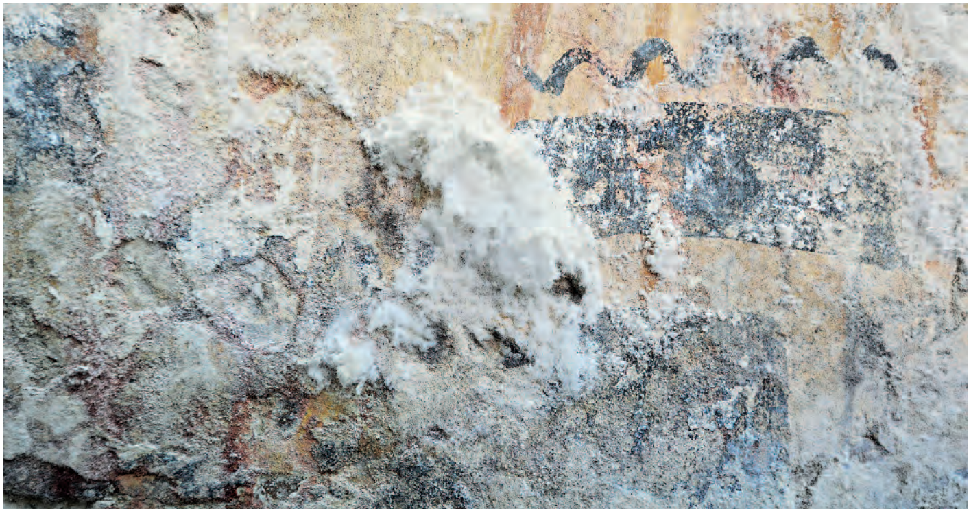
Salt crystals on the surface of a wall painting, no. 8 Universităţii Street, Cluj-Napoca (Romania), 2002; Photo: 2015, UAD (Adrian Rauca)
