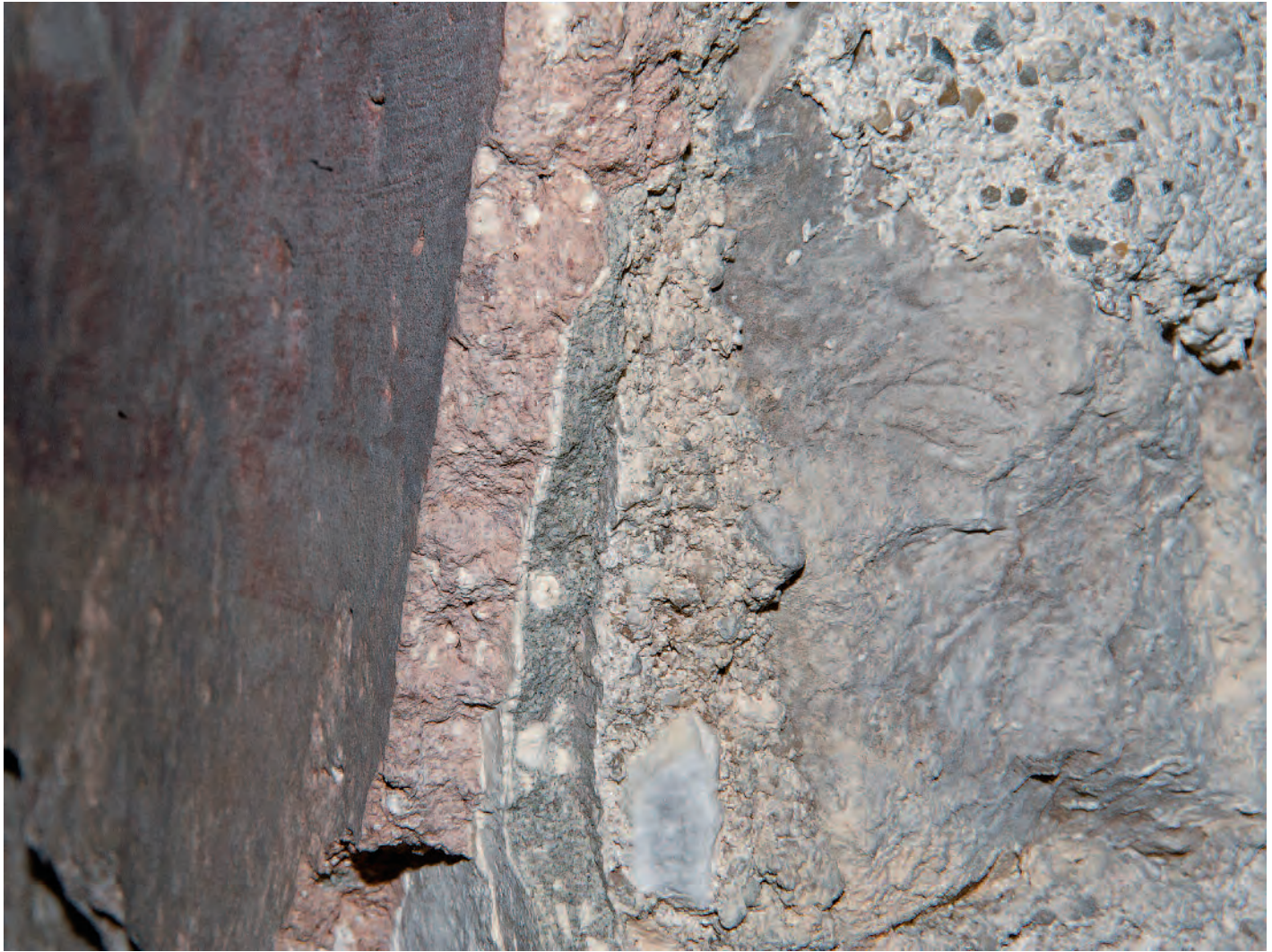
Plaster layers (detail), Dubrovnik Cathedral (Croatia) 10/11th century; Photo: 2011, HRZ (Katarina Gavrilica)
