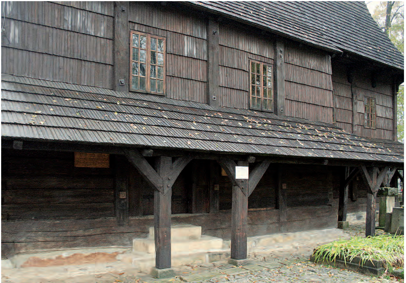
Façade and roofs with wooden shingles, Church of Saint Leonard, Lipnica Murowana (Poland), 15th century; Photo: 2008, UAD (Adrian Rauca)
