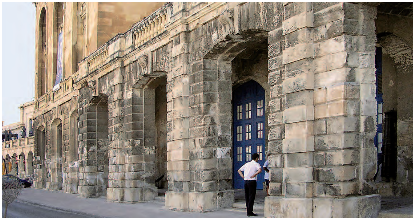
Blackened building due to air pollution (main façade, lower storey in Coralline Limestone), Maritime Museum (Old Naval Bakery), Birgu (Malta), 1842-1845; Photo: 2008, UM (JoAnn Cassar)
