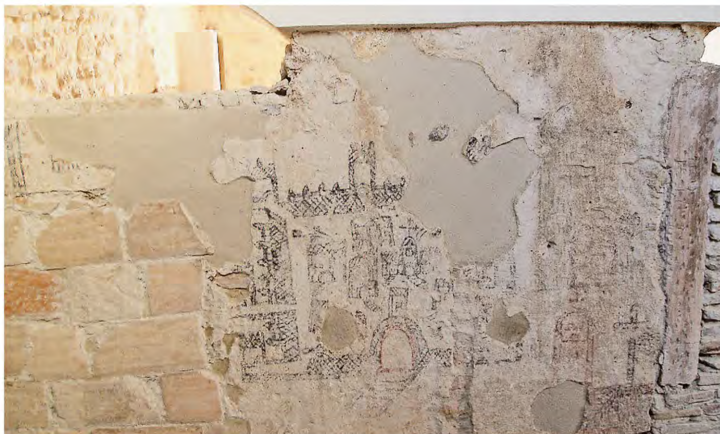
Lacunae infilled in a lower plane than surrounding plaster, Palau de la Vila, Ontinyent (Spain), 19th century; Photo: 2008, UPV (Pilar Soriano Sancho)
