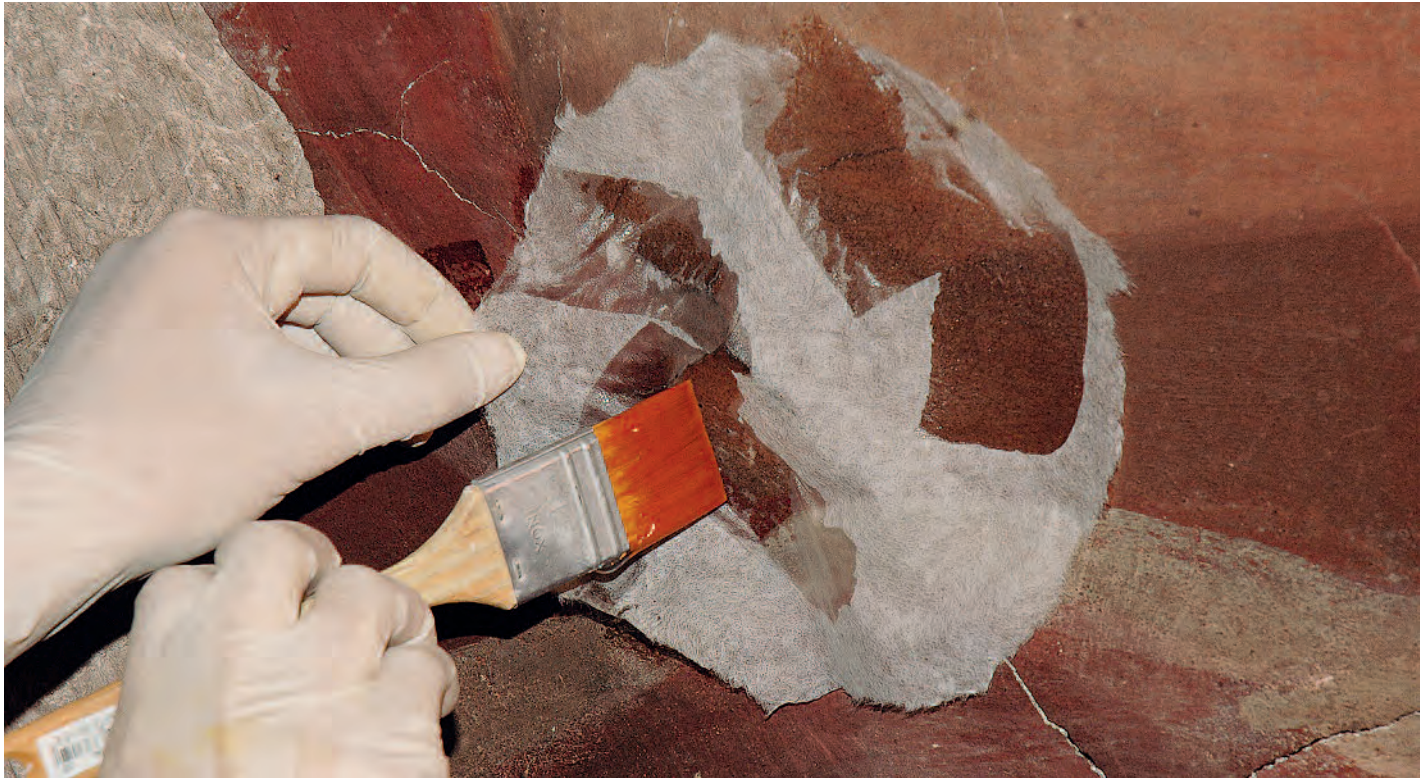
Application of a consolidant, wall painting by Antonio A. Palomino/ Guilló, Church of Santos Juanes, Valencia (Spain), 1698-1700; Photo: 2009, UPV
