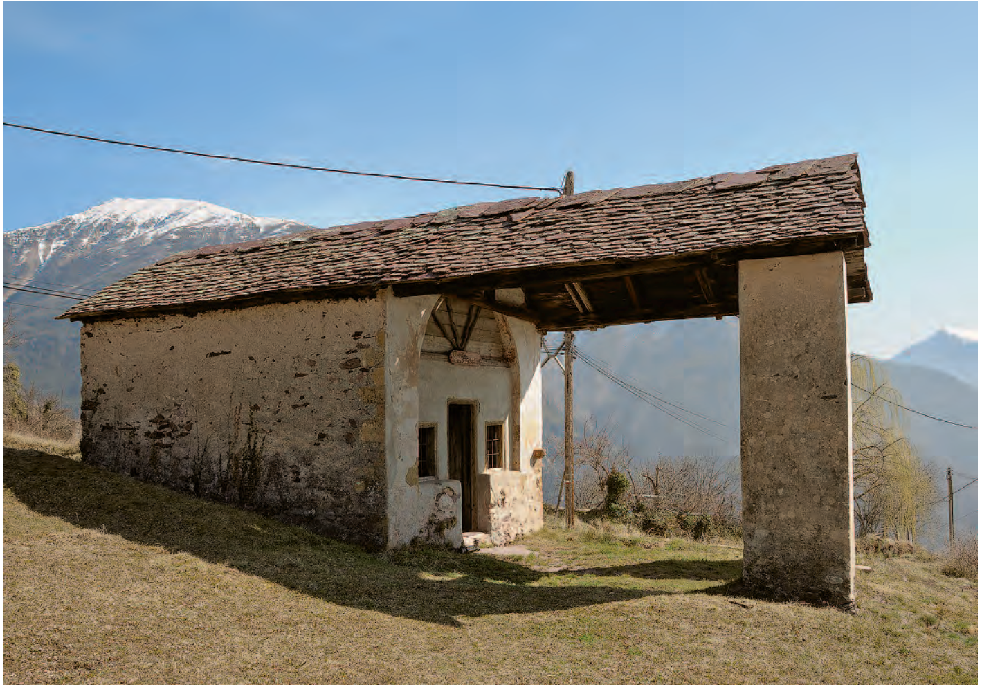
General view of the context (vegetation and ground topography), Chapel of Saint Sébastien, Roure (France), 15th century; Photo: 2011, CICRP (Jean-Marc Vallet)
