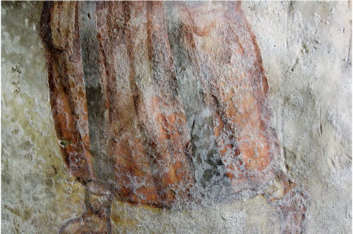
White salt efflorescence, Roman tomb, Silistra (Bulgaria), 4th century AD; Photo: 2014 (Stefan Belishki)
