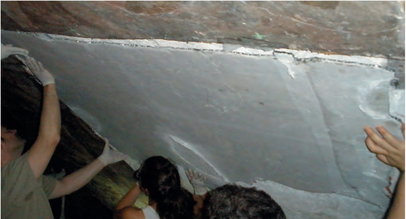
Transfer of a wall painting by Antonio A. Palomino/ Guilló, after its restoration, to its original place: Church of Santos Juanes, Valencia (Spain), 1698-1700; Photo: 2009, UPV (Pilar Soriano Sancho)
