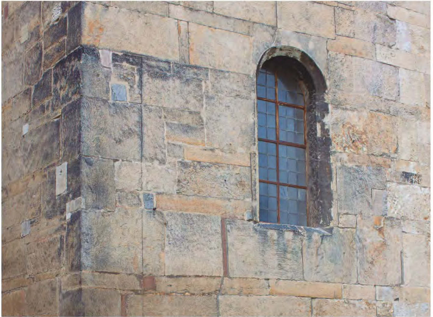
Unrendered masonry surface, Church of St. Michael, 11th century; Photo: 2010, HAWK (Clemens Kappen)
