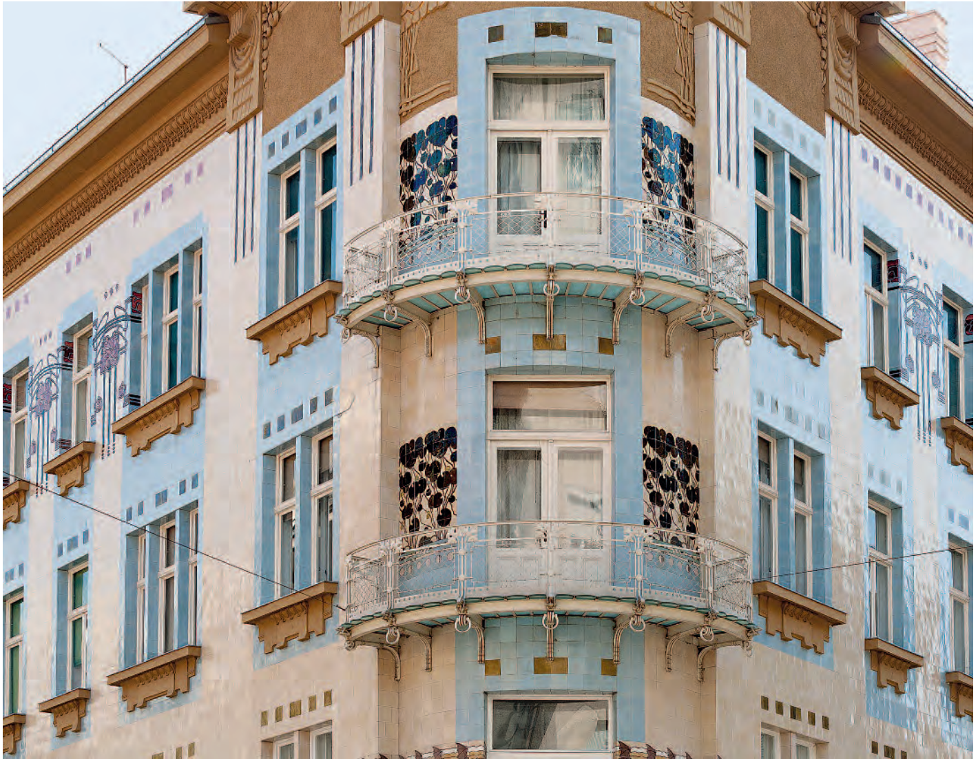
Façade with glazed tiles, Kallina House, Zagreb (Croatia), 1903/04; Photo: 2011 (Branimir Kolarek)
