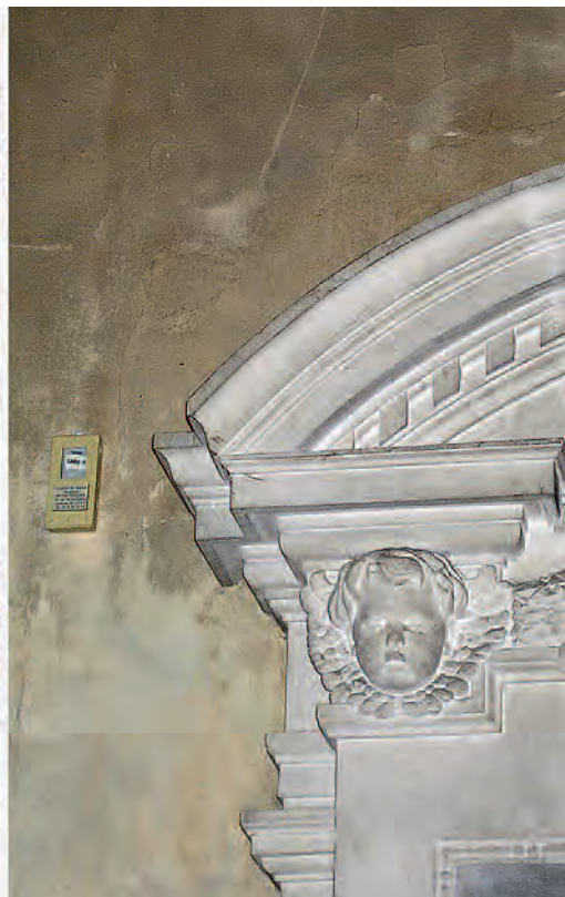
Relative humidity and temperature monitoring, Chapel of Saint Lazare, Aix en Provence Cathedral (France), 12-16th century; Photos: 2000-2004, CICRP (Jean-Marc Vallet)
