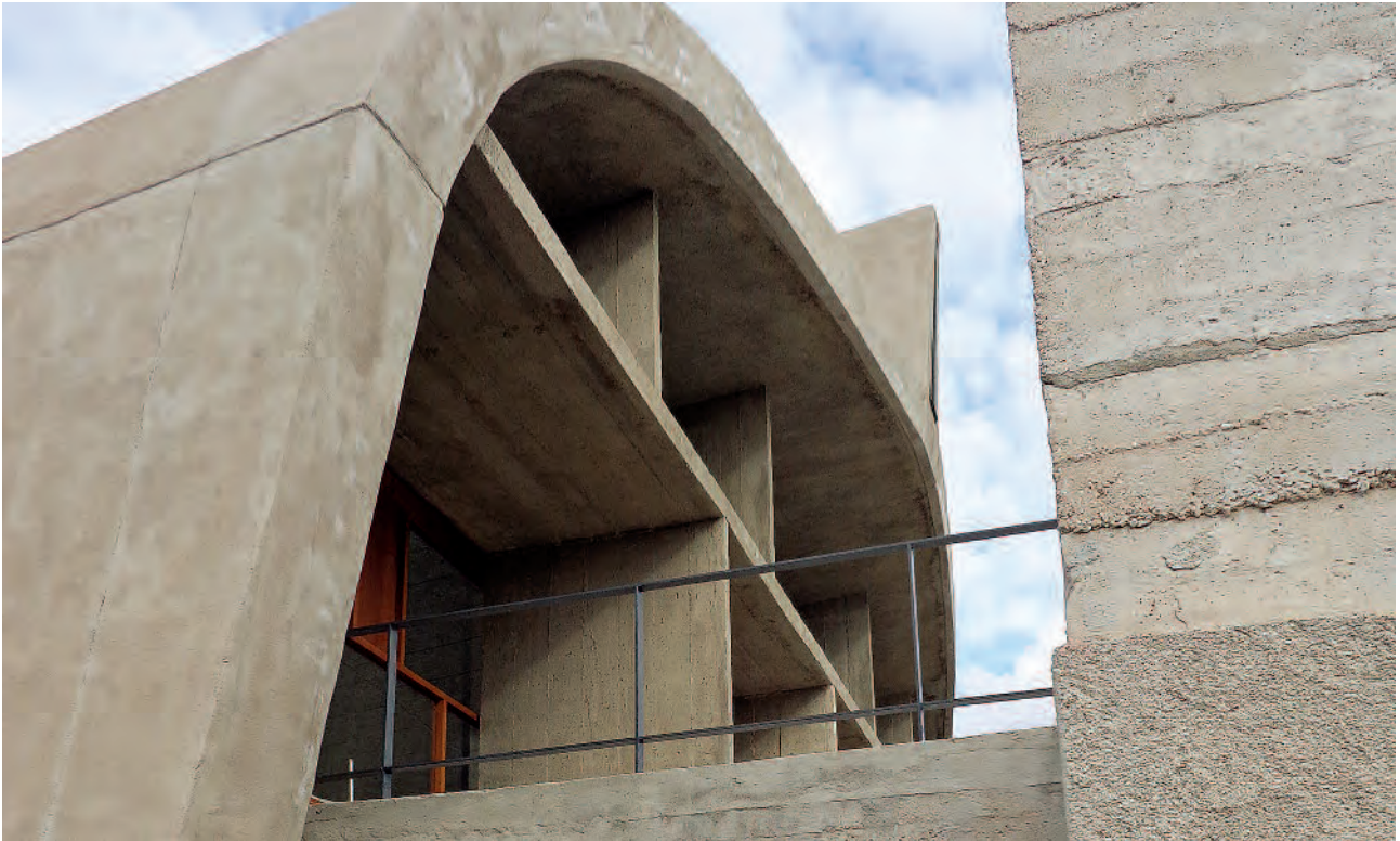
Different concrete surface finishes, La Cité Radieuse by Le Corbusier, Marseille (France), 1952; Photo: 2015, RPS (Dörthe Jakobs)
