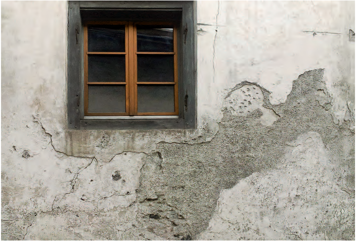
Plaster layers with final render above, historic building, Santa Maria Val Müstair (Switzerland); Photo: 2015, HAWK (Angela Weyer)
