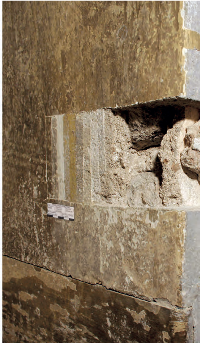
Areas of uncovering, showing successive superimposed paint layers, in a show flat, La Cité Radieuse by Le Corbusier, Marseille (France), 1952 (left); similar uncovering of layers of paint and plaster for an investigation, Church of Saint Nicholas, Ribița (Romania), 15th century (right); Photos: 2015, CICRP (Odile Guillon), 2014, UAD (Adrian Rauca)
