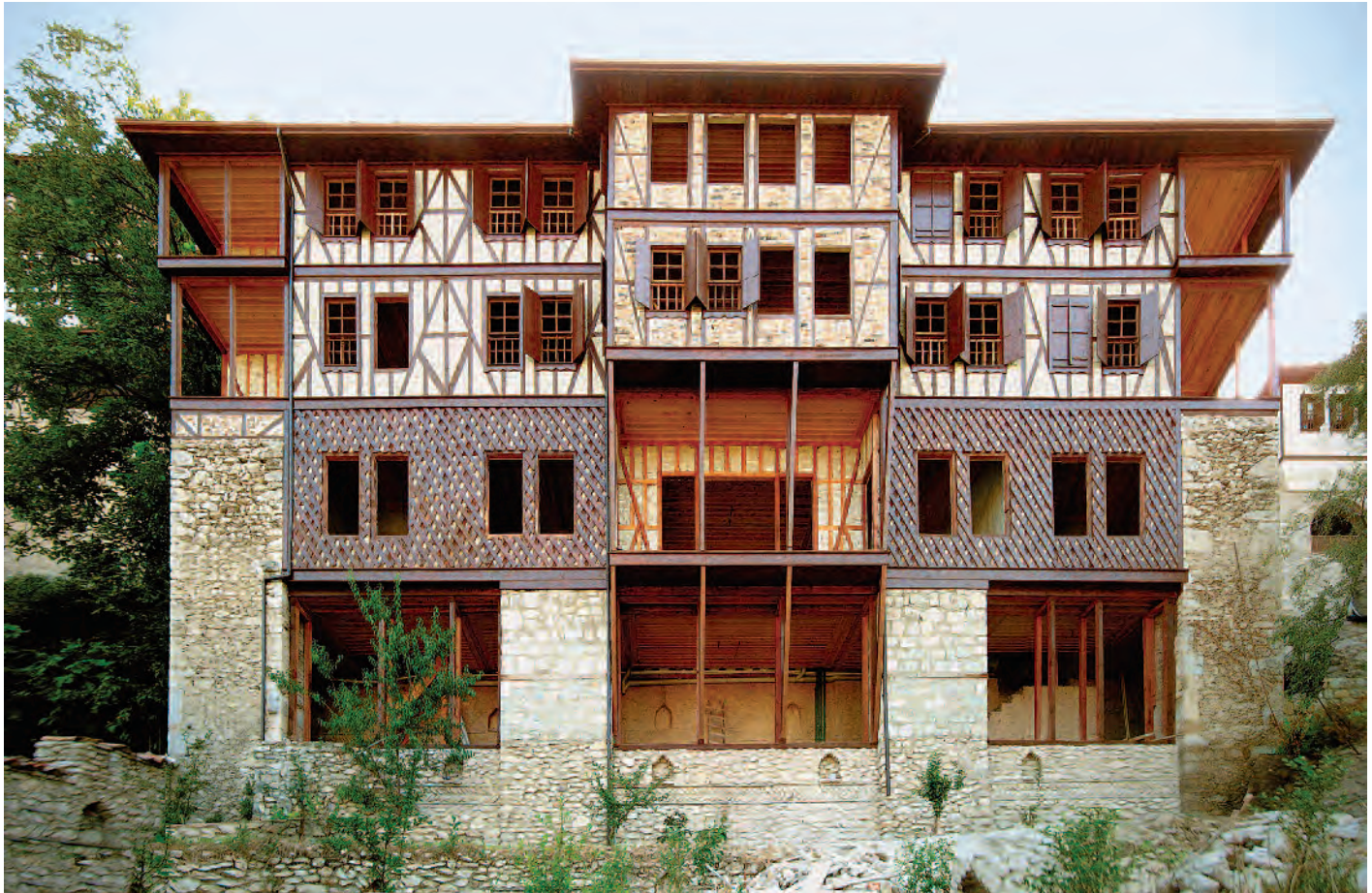
Multistorey half-timber construction, reconstruction of Old Greek Bath House, Safranbolu (Turkey), 19th century; Photo: 2008 (Randolph Langenbach)
