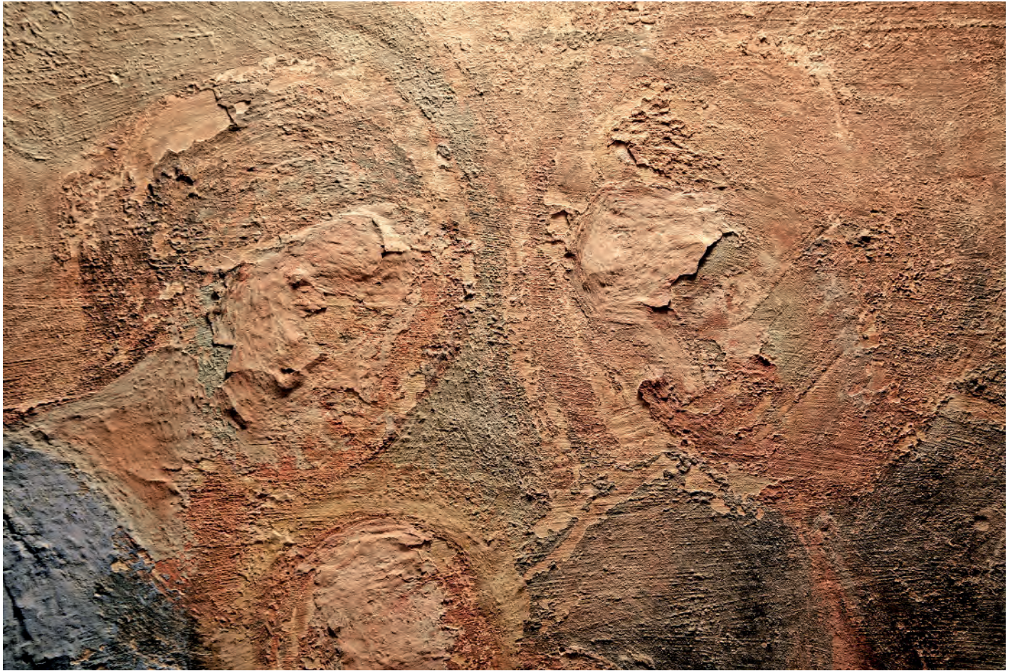
Partly detached paint layer, Franciscan Monastery, Dubrovnik (Croatia), 18/19th century; Photo: 2009, HRZ (Katarina Gavrilica).
