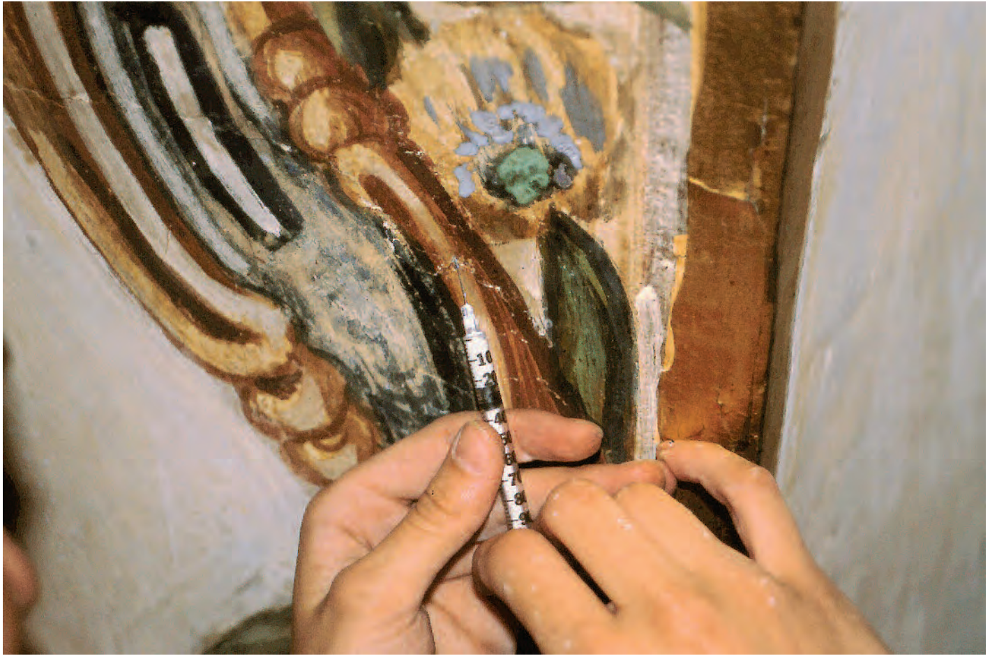
Injection of an adhesive into a wall painting, Church of San Roque, Oliva (Spain), 20th century; Photo: 2009, UPV
