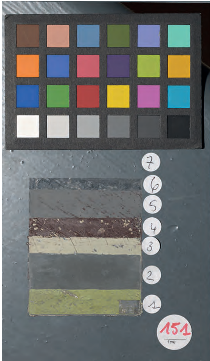
Areas of uncovering, showing successive superimposed paint layers, in a show flat, La Cité Radieuse by Le Corbusier, Marseille (France), 1952 (left); similar uncovering of layers of paint and plaster for an investigation, Church of Saint Nicholas, Ribița (Romania), 15th century (right); Photos: 2015, CICRP (Odile Guillon), 2014, UAD (Adrian Rauca)
