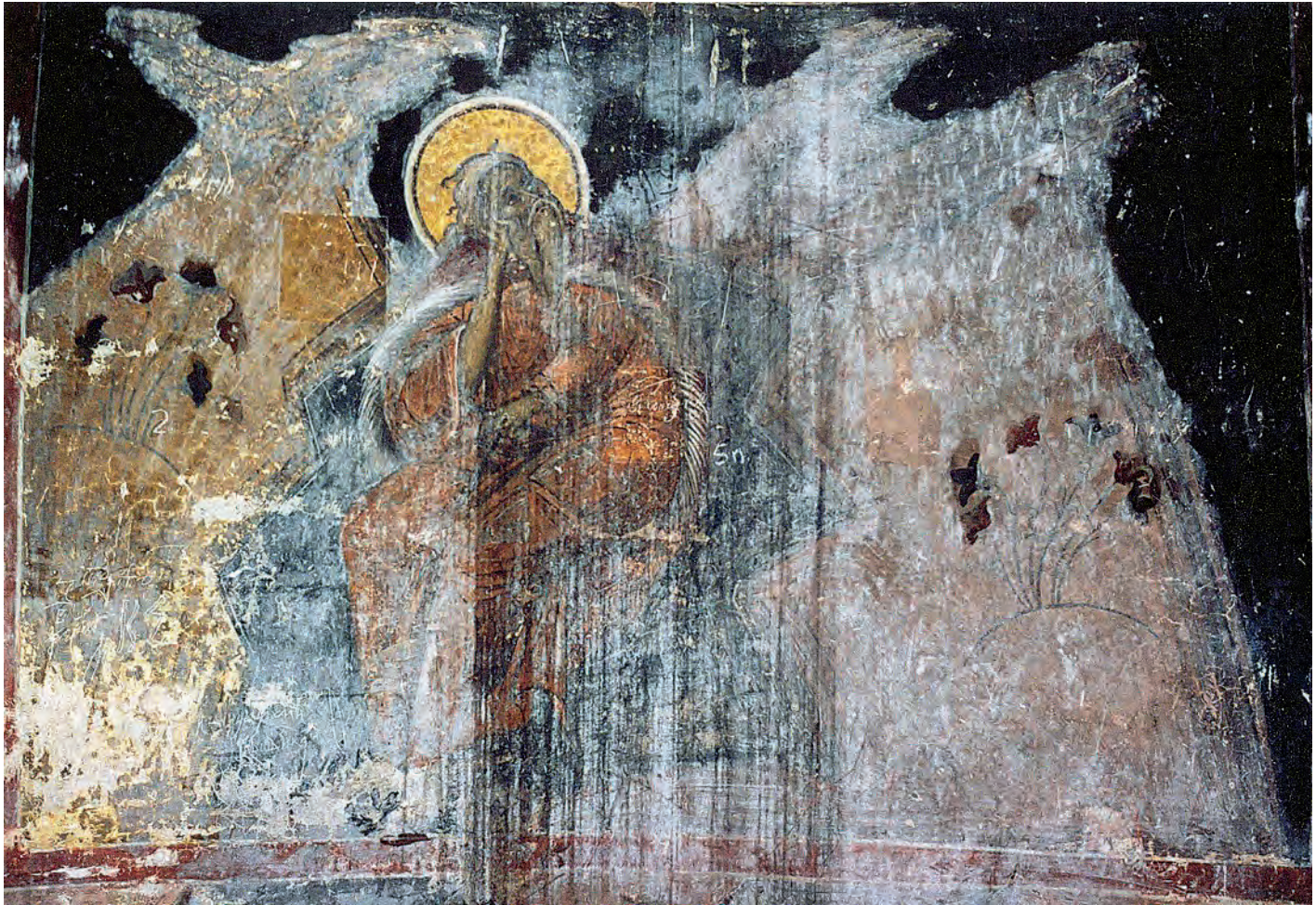
Water drip marks, Moldovița Monastery (Romania), 1532; Photo: 2003, UAD (Theo-Sandu Mureșan)
