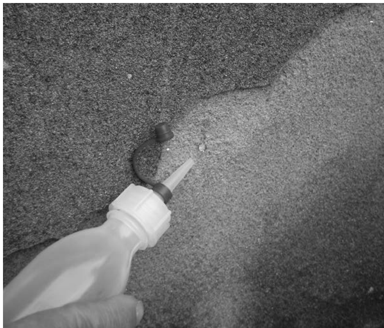
Figure 1. Water drop test performed on a water repellent surface (Photo Christine Blauer).
