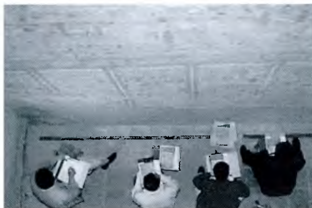
Figure 7. Condition recording, Cave 85, Mogao Grottoes [Photo: Leslie Rainer].
