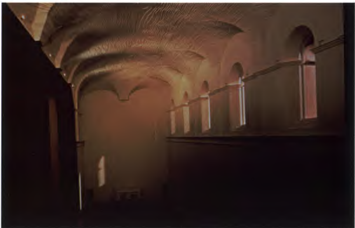
Figure 3. Interior of the 1:20 scale model of the Sistine Chapel, showing the ceiling's contour lines based on the photogrammetric survey.
